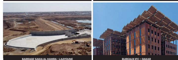
BARRAGE SAKIA AL HAMRA - LAAYOUNE
